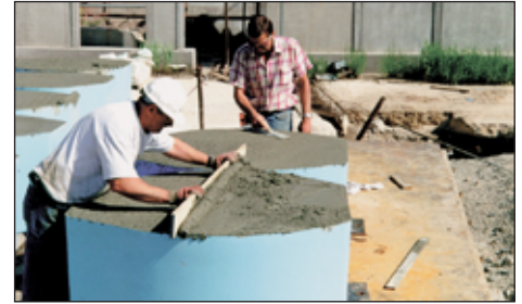
Step 6: Settle and level base of fiberglass shell, allow concrete to cure
