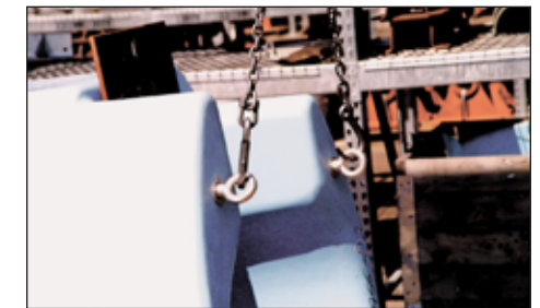
Step 9: Once concrete filled basin is resting in a vertical position, switch lifting rigging from single hoist plate* / fastout device** to double lifting eyes. Do NOT lift basin! Slowly lower basin to rest upright on level ground***
